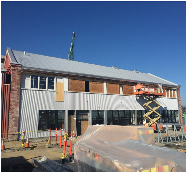
Construction taking place on WETA's new Mare Island Ferry Facility
